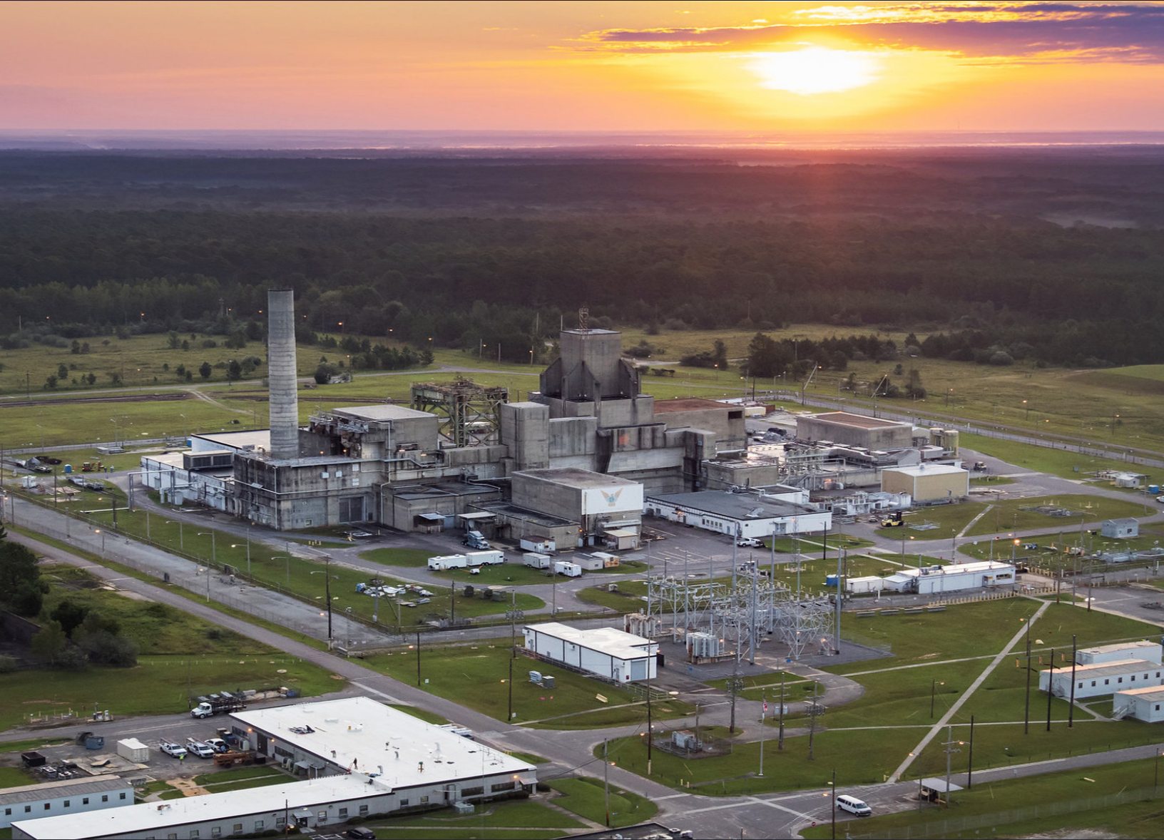
Photo Credit: U.S. Department of Energy
