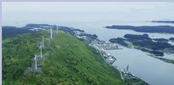
Wind turbines in Kodiak, AK. Image Source: ABB Group.
