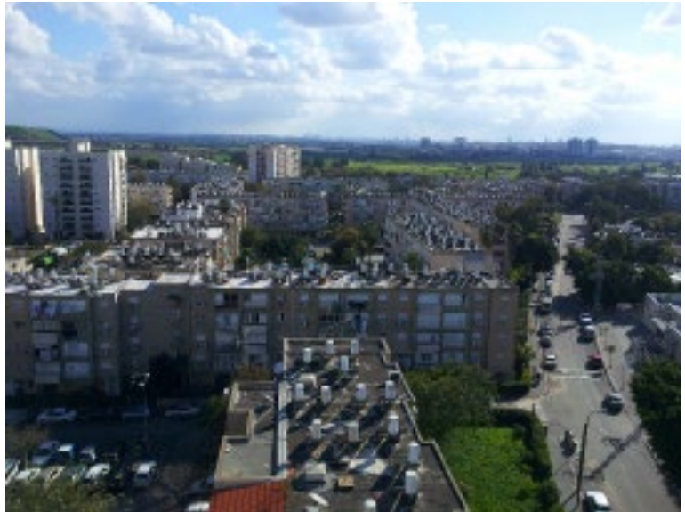
Tel Aviv, Israel. Note the Rooftop Water Heaters
