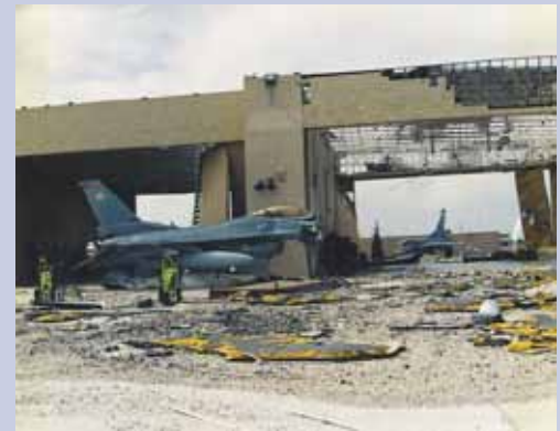
Damage to Homestead Air Force Base after Hurricane Andrew
